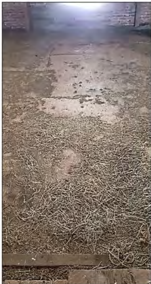
Plywood Flooring at West End
