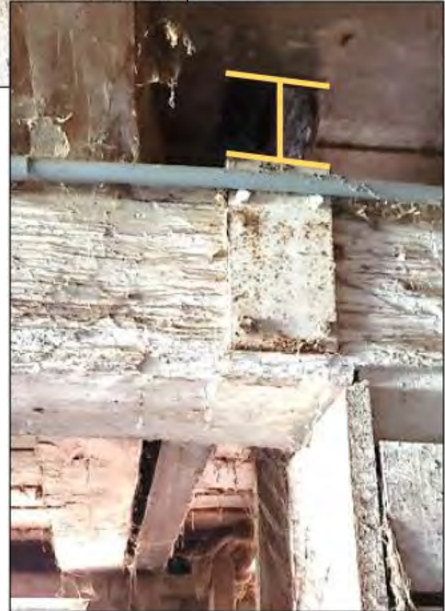
Inserted Steel Beams Inside Barn
