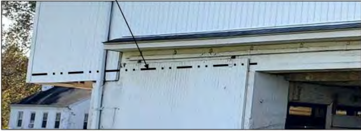
Location of Steel Beams
