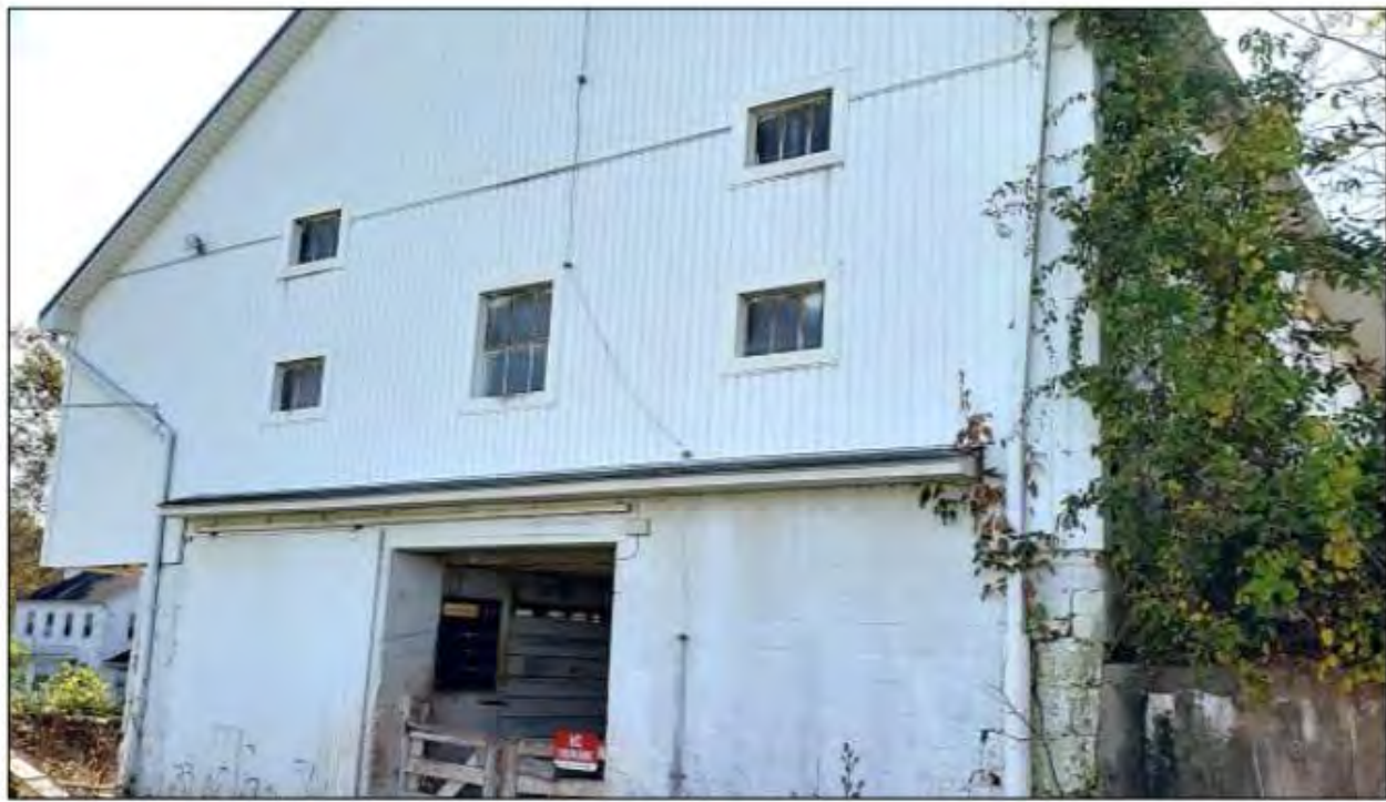
Concrete Block End of Barn
