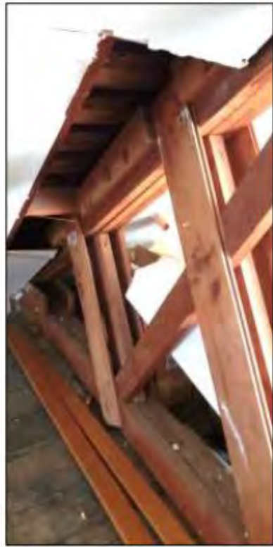
Truss constructed of dimensional lumber supporting roof, with iron turnbuckle supporting lower chord.
