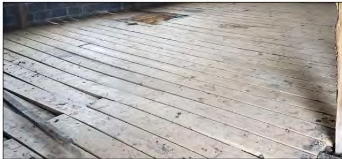
Dimensional Lumber Flooring at East End
