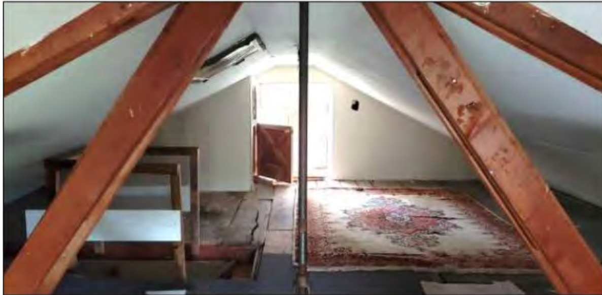
Truss constructed of dimensional lumber supporting roof, with iron turnbuckle supporting lower chord.
