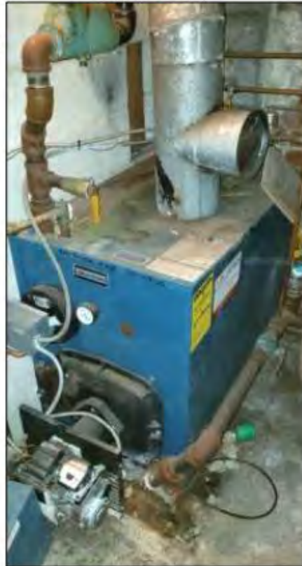
Oil Fired Boiler
